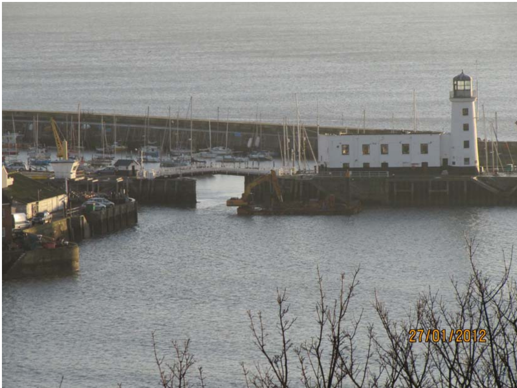
Figure 5 – Dredging of the Approach Channel to Old Harbour (January 2012)
