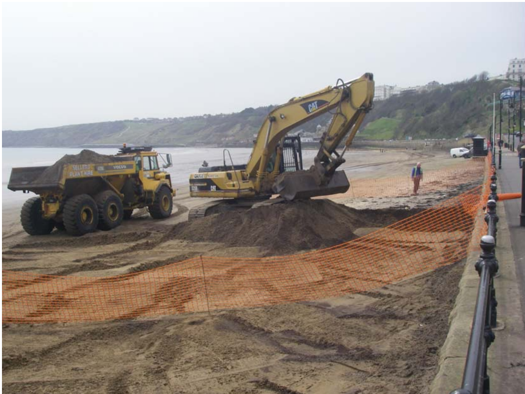
Figure 2 – Sand excavation in progress (2008)
