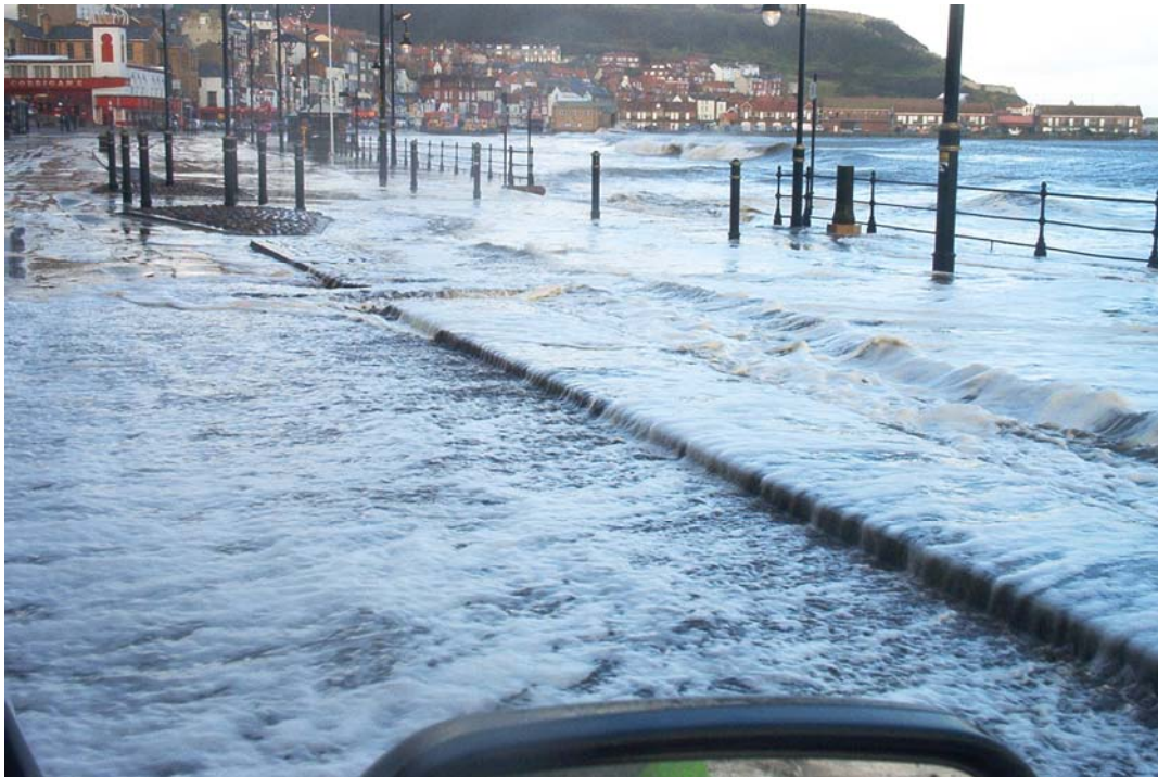
Figure 4 – Flooding of Foreshore Road due to Wave ‘Ramping’ (20 th March 2007)
